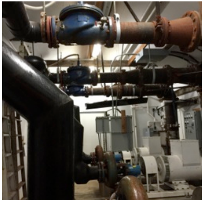
West Hydro building at Port Armstrong. Photo by Bart Watson
